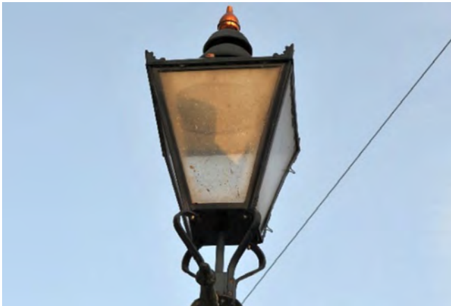
▲ d. Waters Traditional V1BGO. ‘Pot’ optic set within canopy 70 W SON-T (Urbis Abbey, Metcraft Victoria and DW Windsor fittings are all of a similar gas-lantern style).
