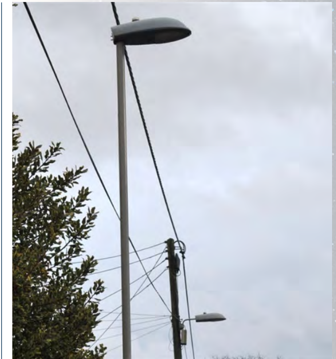
▲ Fig. E4: Philips SGS 252 Flat Glass 70 W CDO Luminaires at Sixpenny Handley (typical column and wood-pole mounting). These types of fittings comply with IDA light control requirements. Colour temperature, however, varies with light source, with most in this area being CDO 4000 K.
