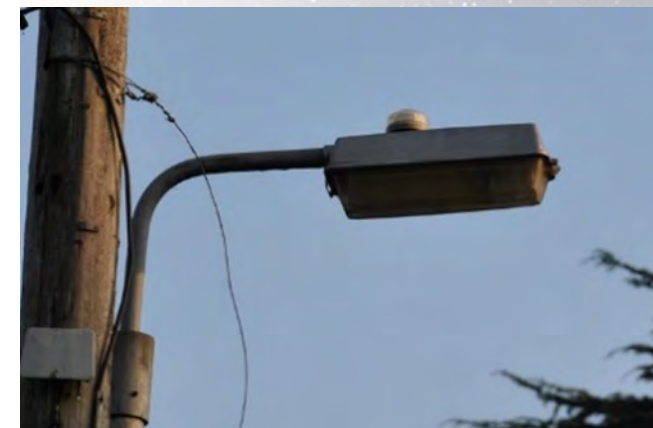
▲ Fig. E2: Thorn Beta 5 street light: a typical 35 W SOX fitting mounted on wooden electricity distribution pole. (Philips, GEC and others have fittings in very similar deep-bowl refractor-optics style.)
